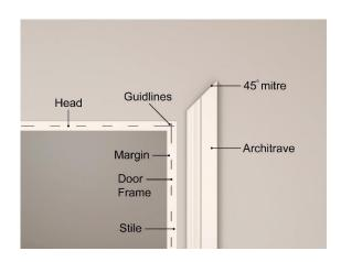
3 Vertically align the architraves to the margin marks on the stile of the door frame. Architraves can either be nailed using 16 gauge nails or Tech 7 MS Polymer based adhesive. Nail holes can be filled using Tech 7 adhesive. Excess adhesive can be easily removed using builder's wipes. If desired, once the filler is dry, a small dab of our touch-up paint may be used to seal the filler.
